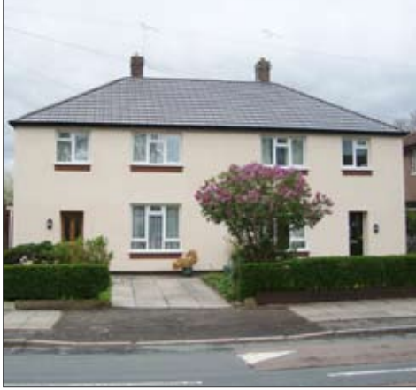
Concrete block property after refurbishment
